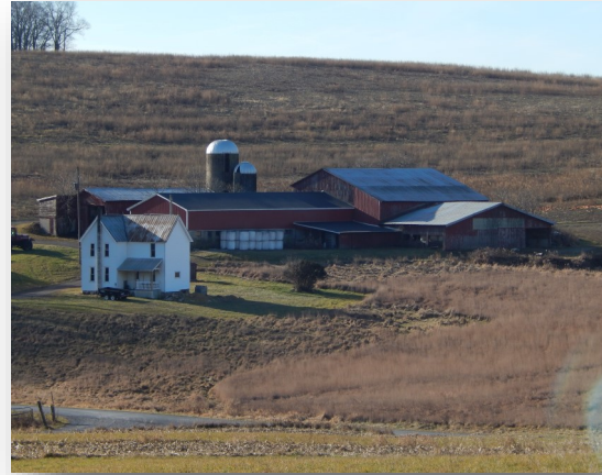
Farm #2 1301 Stoney Batter Road Hughesville, PA
